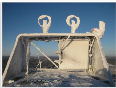
Figure 4: Nacelle cooling affected by snow and ice. Gearbox test bench in OWI-Lab climatic test chamber.
